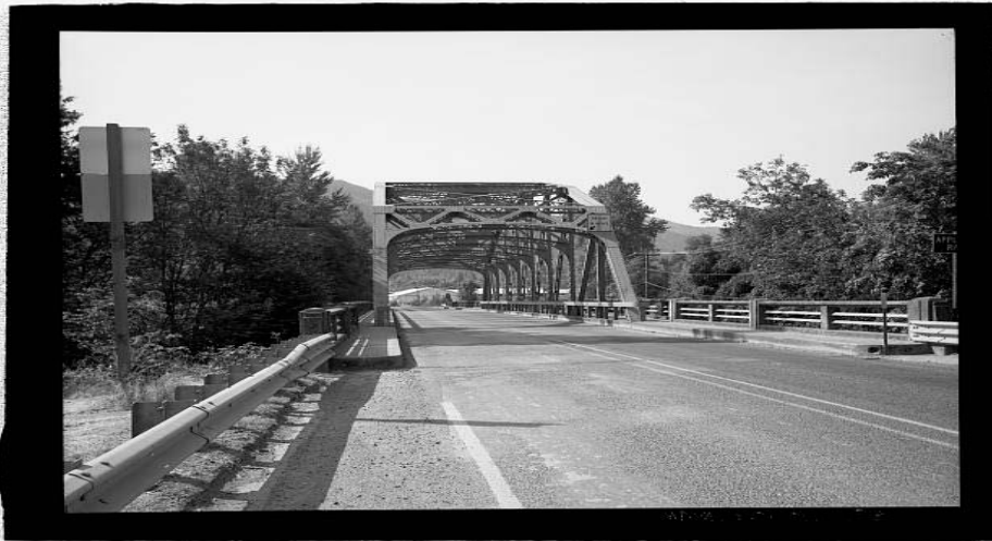
The Applegate (Murphy) Bridge on Highway 238 near Murphy, Oregon was built in 1935 by Glenn S. Paxson. It is a steel truss bridge with Parker through truss construction and spans 450 feet. This was the truss type of construction predominate at the time and is now obsolete. It was replaced by a steel plate girder bridge in 2004.
